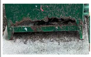
Refuse Container Enclosures – Refuse container enclosures are rusted and missing protective edge banding which can protect against lacerating patrons. Steel ground protrusion nearby is a trip hazard.
