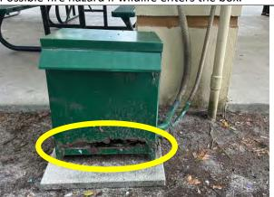
Please consider having all electrical equipment inspected by a licensed professional to determine if the equipment enclosure can be repaired or replaced or if additional shielding is required to prevent access to high voltage equipment.
