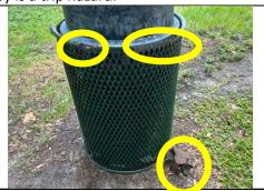
Please consider inspecting all refuse enclosures for corrosion, missing edge banding or other sharp edge hazards and repair as needed. Please consider removing or cutting off the steel ground protrusion to eliminate the trip hazard.
